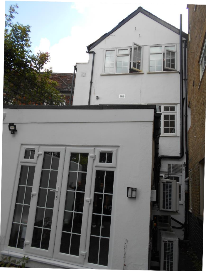
Rear elevation of the listed building with existing location of air conditioning units
