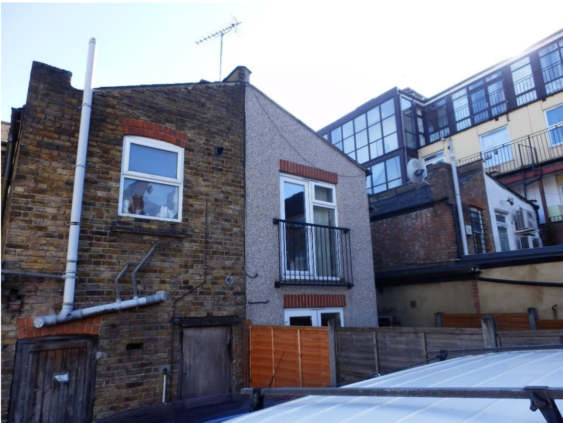
Rear of no. 14
