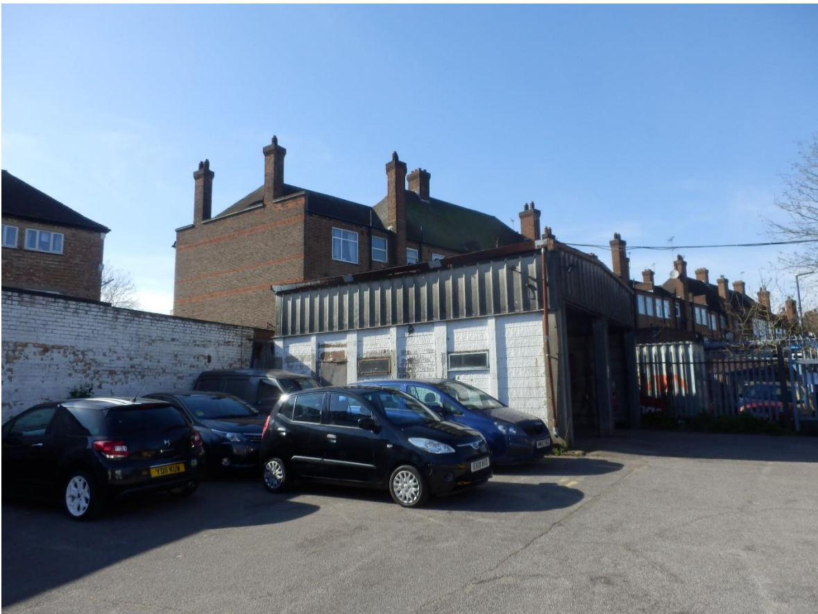
Looking towards rear of shops /flats on Station Road
