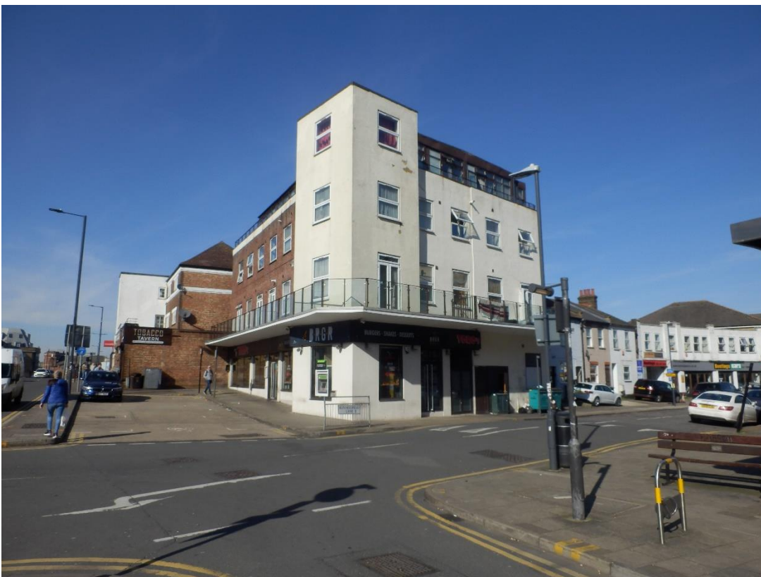
Looking towards site from Station Road
